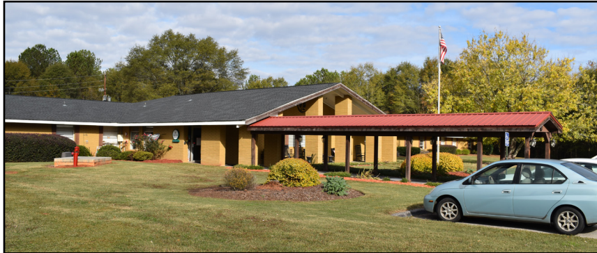
Figure 23. Social Circle Nursing and Rehabilitation Center
